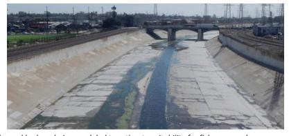
Figure 4-6: Potential future flows following modifications of the channel bed are being modeled to estimate suitability for fish passage (upper right). Soft bottom sections within the Elysian Valley are suitable for fish passage, but are separated from the ocean by concrete bottom sections with flows that are too strong over long distances to allow migration of steelhead (bottom right).
