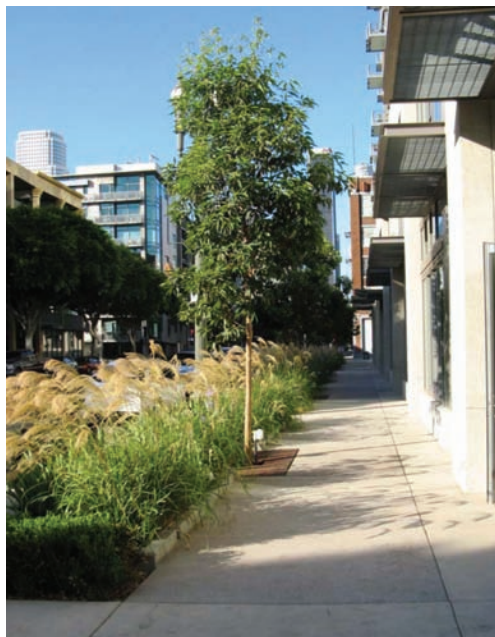
Native vegetation separates the sidewalk and the street, capturing regular urban runoff before it reaches the storm drain system.
