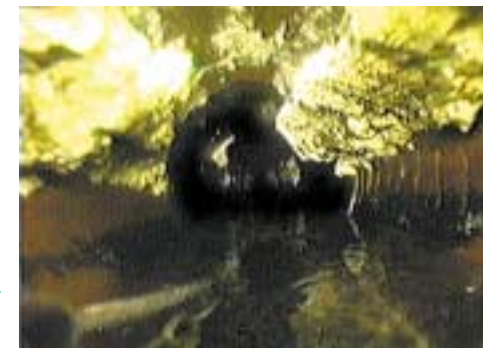
Actual photo taken by remote controlled camera showing grease buildup in sewer pipe interior.
