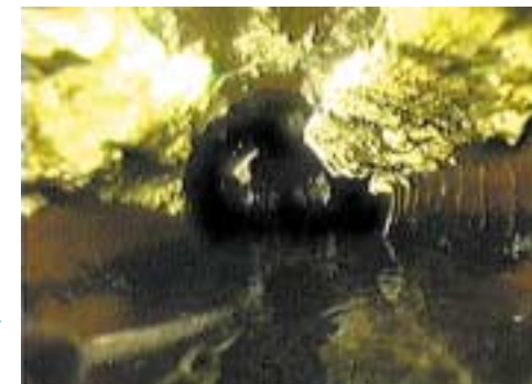
Actual photo taken by remote controlled camera showing grease buildup in sewer pipe interior.
