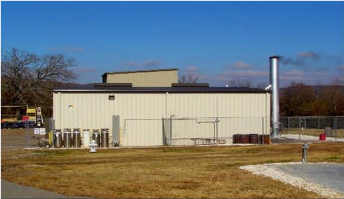
BRI pilot plant processing building; with temporary flare in the background
