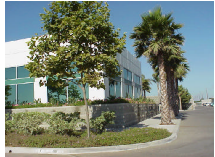
New Transfer Station (Oxnard, California)
