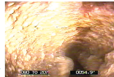
Photo taken via remote controlled camera showing FOG buildup in sewer pipe interior.
